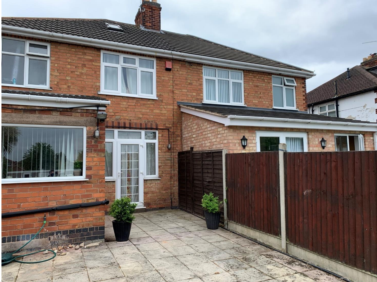
Rear elevation towards 94 Kerrysdale Avenue
