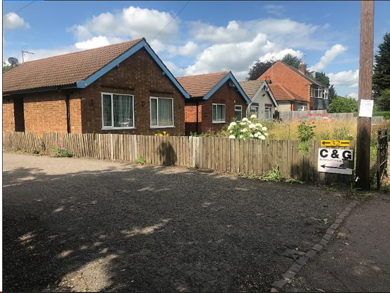
View of front of No 34 & 36
